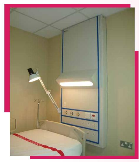
All the front panels can be opened from the front to ease the maintenance work.
